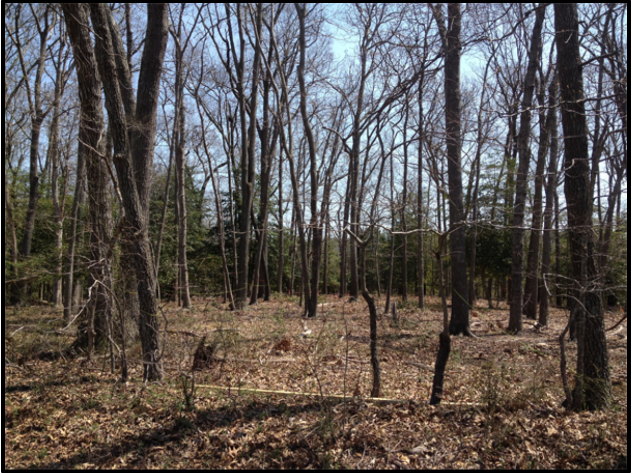
Figure 2. Site before clearing
