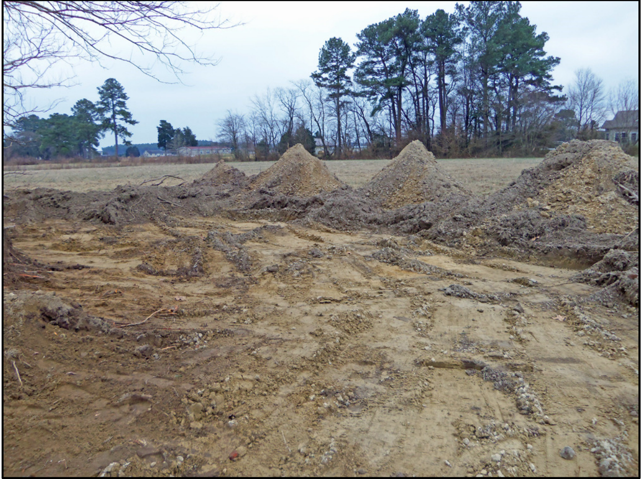
Excavation Outside Limits of Cemetery with No Burials Present
