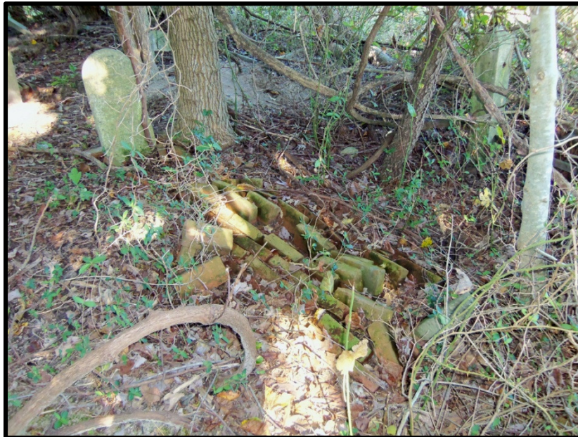
Figure 7. Brick Vault at Surface
